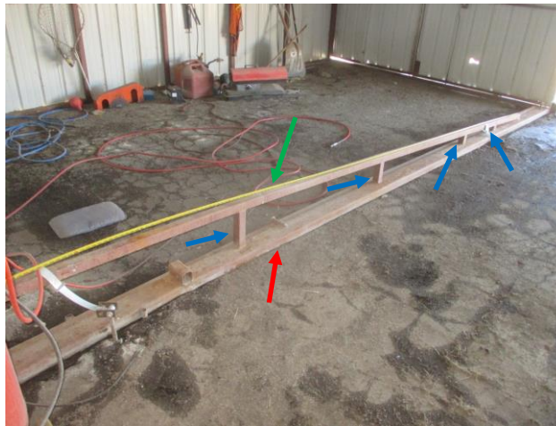
Figure 2. View of right lower frame assembly to be replaced.
