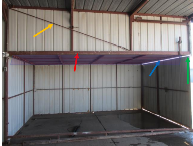
Figure 1. View of a typical upper side wall frame.
