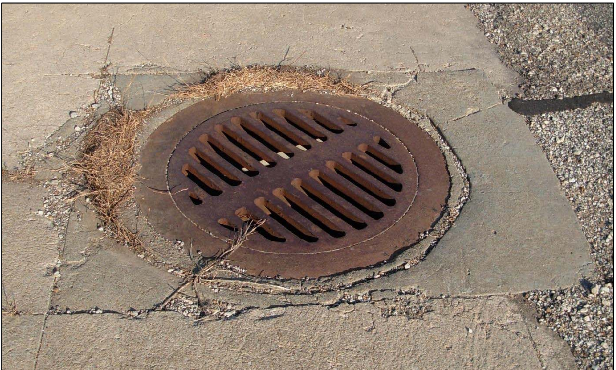
Drive Grate Inlet
