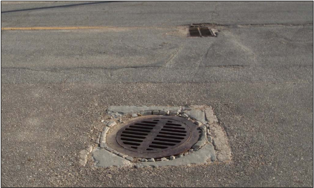
Drive Grate Inlet and Centerline Grate Inlet
