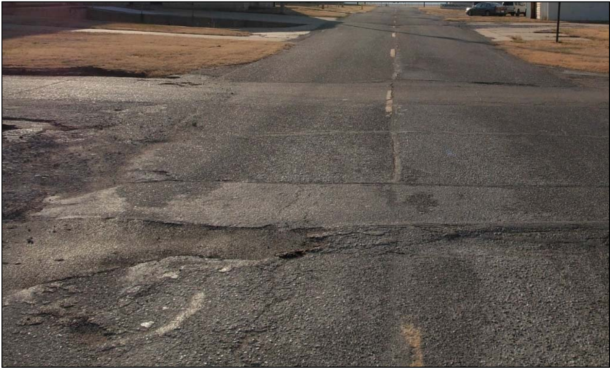
Beechcraft Road Pavement Failure
