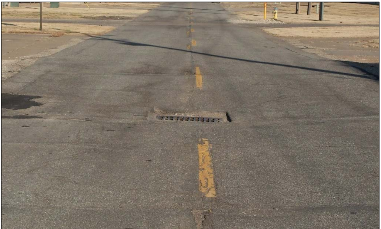
Beechcraft Road with Centerline Grate Inlet
