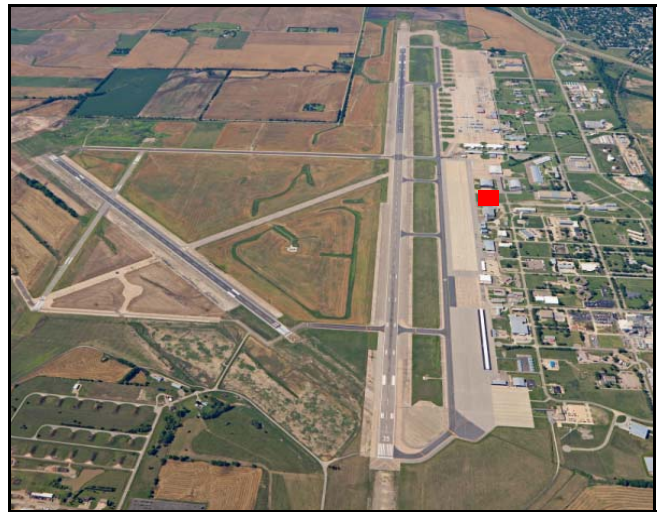
The development of the SLN Aviation Service Center is a partnership of the Salina Airport Authority, City of Salina, Saline County, Salina Area Chamber of Commerce and the Kansas Department of Commerce.
