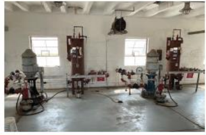
FUEL PUMPHOUSE TO BE DEMOLISHED
