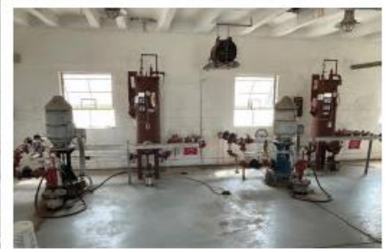
FUEL PUMPHOUSE TO BE DEMOLISHED
