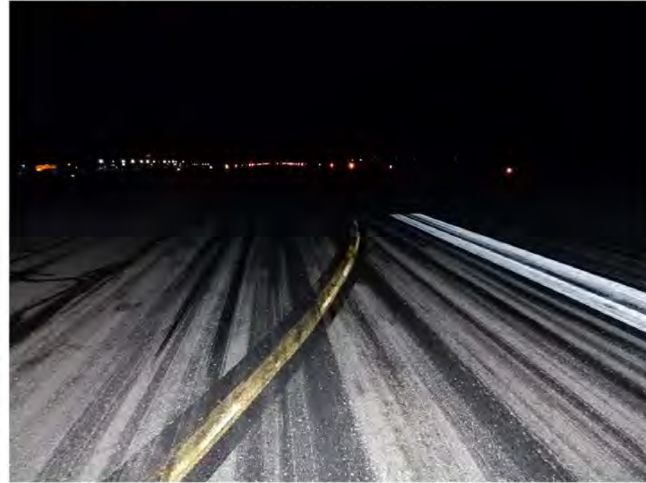
Taxiway Bravo Centerline – (Lead-off/Lead-on for RWY 17-35)
