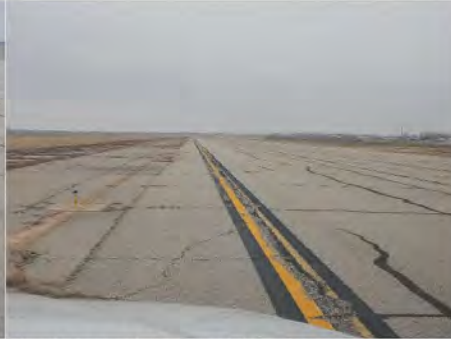
Taxiway Alpha – Edge Marking
