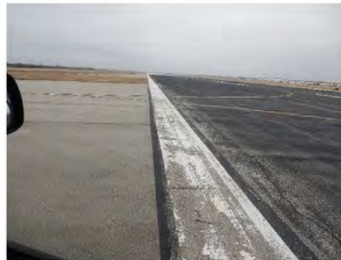
Runway 17-35 – Edge Marking @ E
