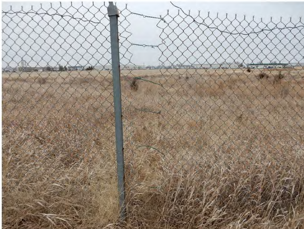
Airport Perimeter Fence
