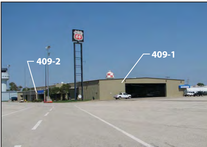
409-1 - Hangar/FBO; 409-2 - FAA Sector Field Office
