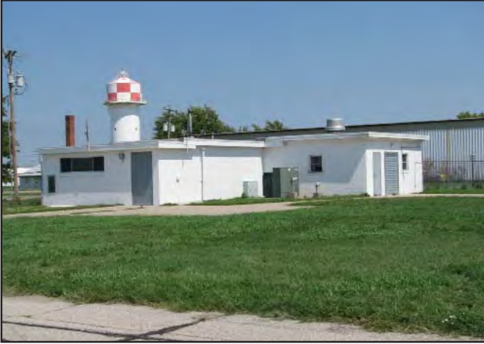
500E - Airfield Electrical Vault
