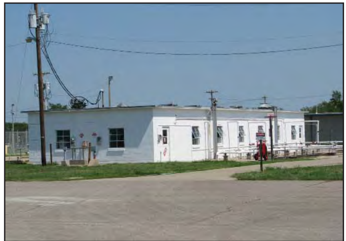
305 - AvFuel Pump House
