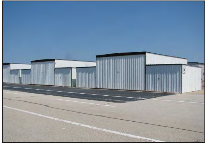
E - Box Hangars
