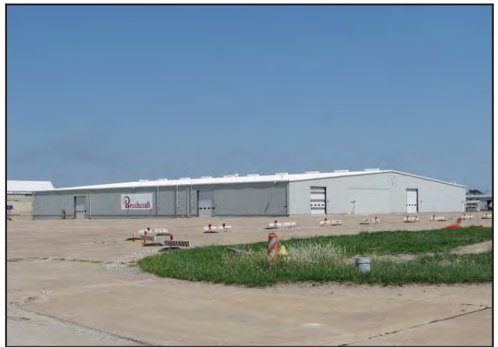
614 - SAA Maintenance & Operations
